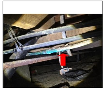
Water dripping from compromised copper pipe. This is only a small leak problem.
