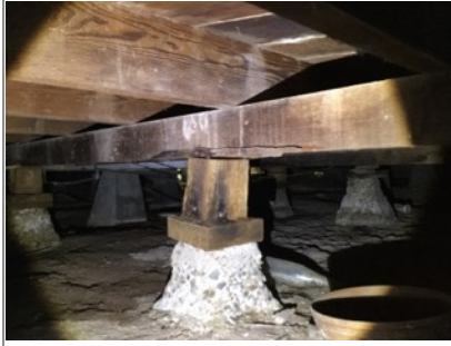
Concrete pier in one of the wet zones. It is eroding.
