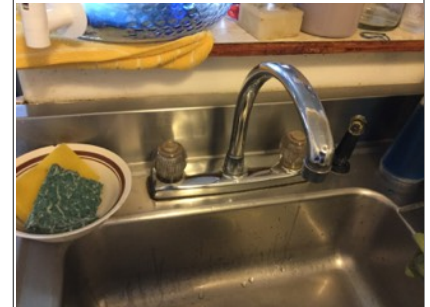
Faucet does not function well. Have to turn to just the right spot to shut off.
