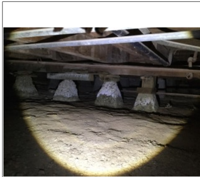
Another area of wet and eroding piers.
