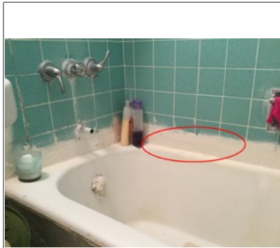
Bathtub has sank and is not level. I recommend repair by a qualified tradesman.
