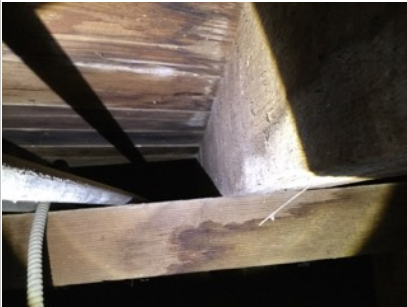
View of girder, floor joist, and subfloor. No defects are noted in this picture.
