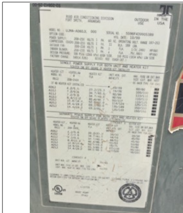
Rudd, 5 ton, 1999, Maximum breaker allowed is: 60 a
