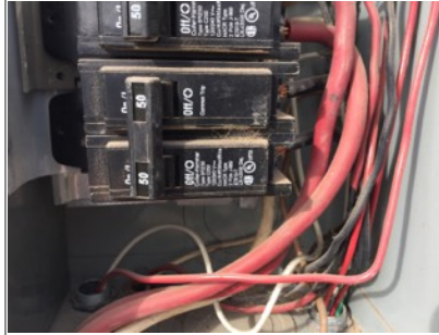
AC breaker 50 a. Ok AC is not grounded. The ground wire is there to prevent shock and maintain safety. This is a safety hazard.
