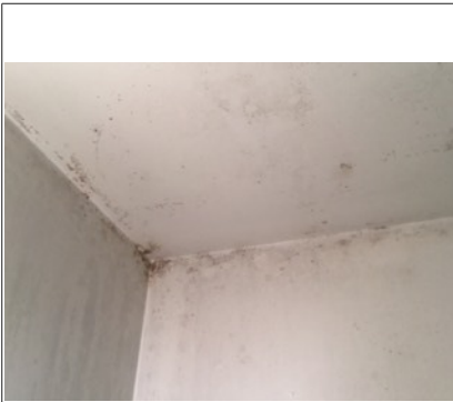
Ceiling and wall are discolored. I recommend more ventilation.
