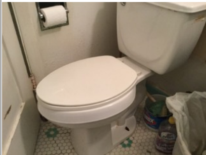
Toilet is loose. Floor has damage.
